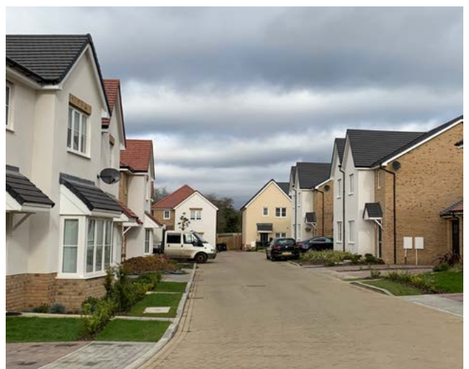
Shared surfaces to streets and minimal use of tarmac. A mix of render, buff brick and weatherboard.
